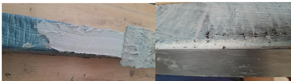
Figure 4. Application of the carbon fiber plate composite material over the fabric
