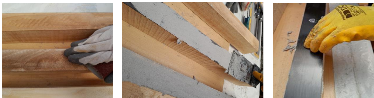
Figure 2. Preparing the beams for consolidation with carbon fiber plate
